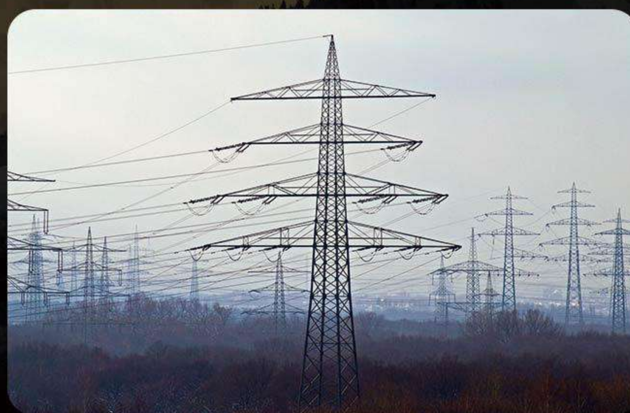
Power line surveying
